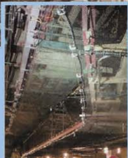
More than 440,000 sq. ft. of safety netting was installed under and around 20 miles of steel track that manage checked baggage at Denver International Airport.
