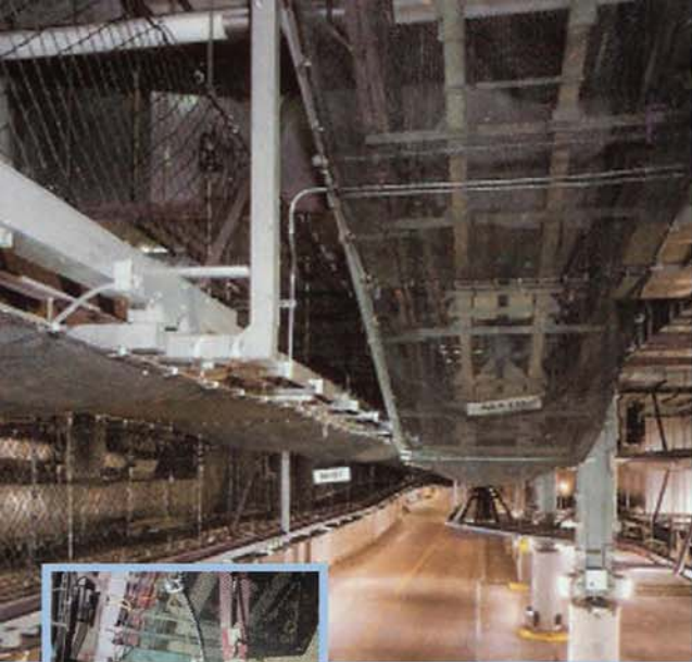
More than 440,000 sq. ft. of safety netting was installed under and around 20 miles of steel track that manage checked baggage at Denver International Airport.
